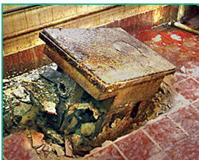
Rusted Steel Grease Interceptor Typical life expectancy is 5 years.
