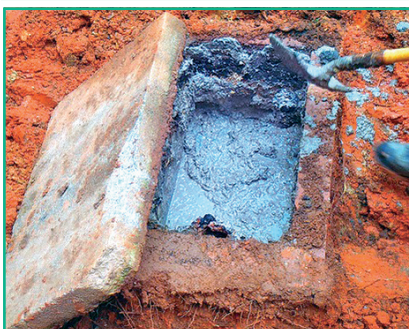
Corroded Concrete Interceptor Typical life expectancy is 10 years.
